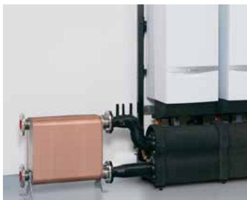
Plate heat exchanger installation
