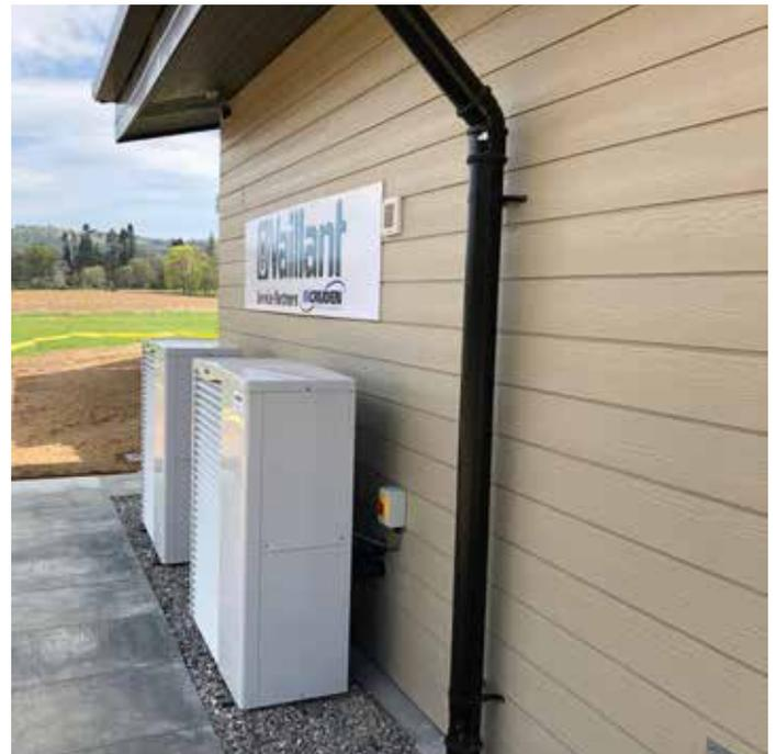
The use of the Vaillant heat exchanger module also contributed to cost savings in the form of saving on glycol required for the heating system. The system is complemented by the Vaillant VRC 700 weather compensating system control which intelligently communicates with all Vaillant appliances.
