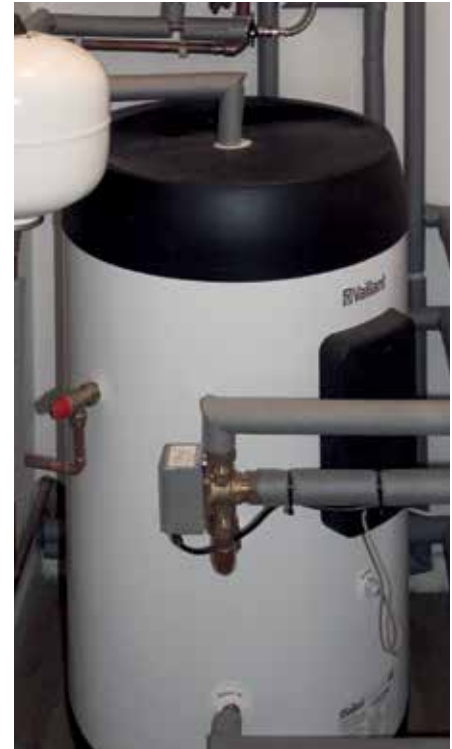
150 litre uniSTOR hot water cylinder
