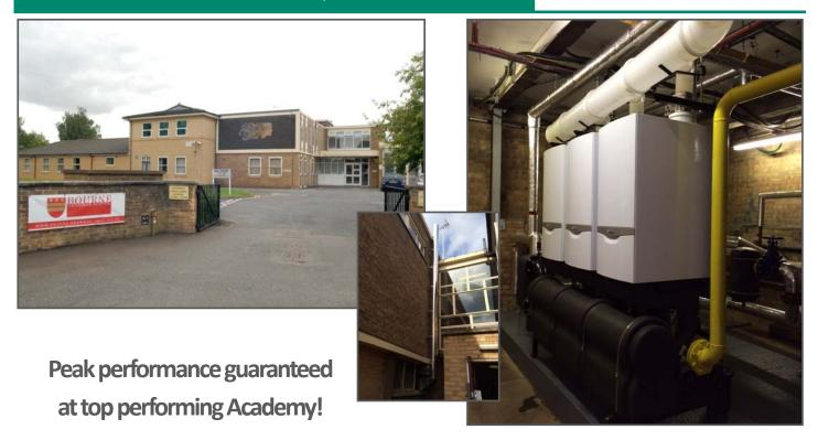
Ageing Hoval boilers were replaced with three ecoTEC 120kW boilers together with a Vaillant VCR 103 boiler mounting frame with hydraulics and insulation for ease of installation.
